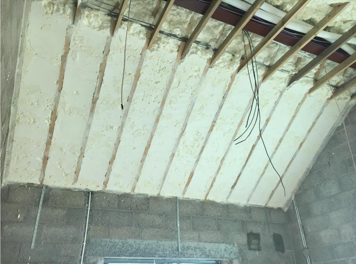
Figure 2 - close-up showing the Product detailing around steel RSJ and dwarf partition wall; prior to dressing back flush with the rafters
